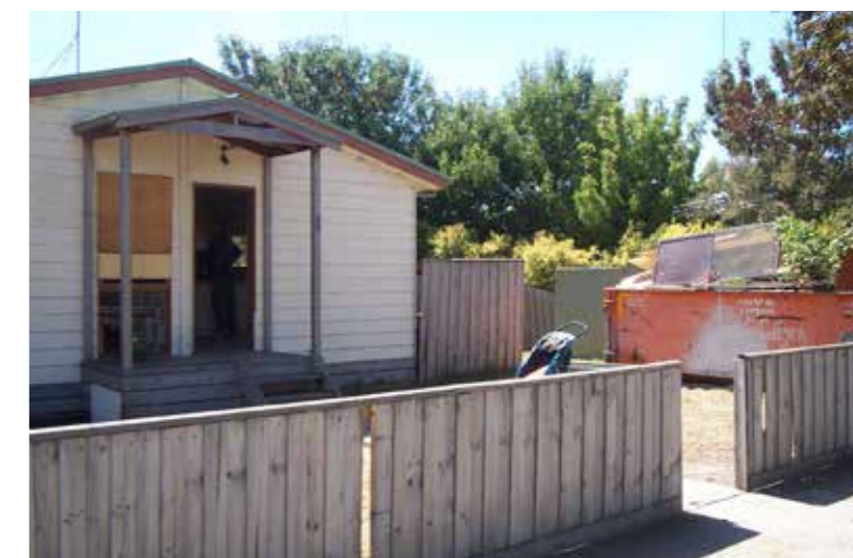
BYAS partnered with not-for-profit organisation, Kids Under Cover, to provide relocatable bungalows and units, such as this one, for homeless young people. By 2006 BYAS was managing 10 Kids Under Cover properties in Geelong and Colac.
